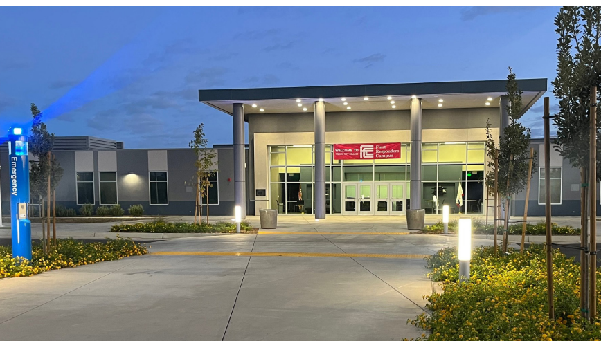
First Responders Administration Building (October 2023).
