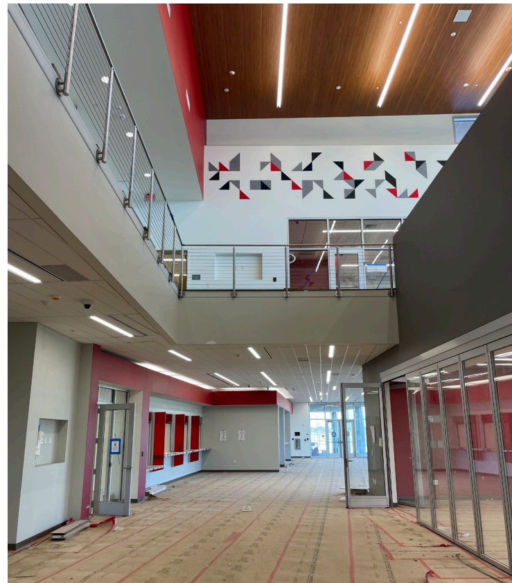
West Fresno Academic Building Lobby (July 2023).
