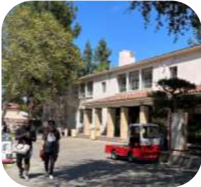
Student Center, in fair condition
