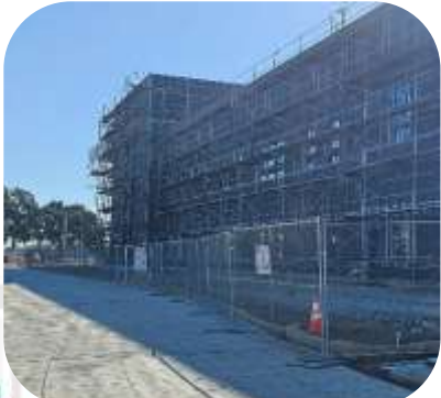
Science Building, in construction
