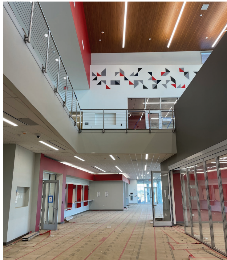
West Fresno Academic Building Lobby (July 2023).
